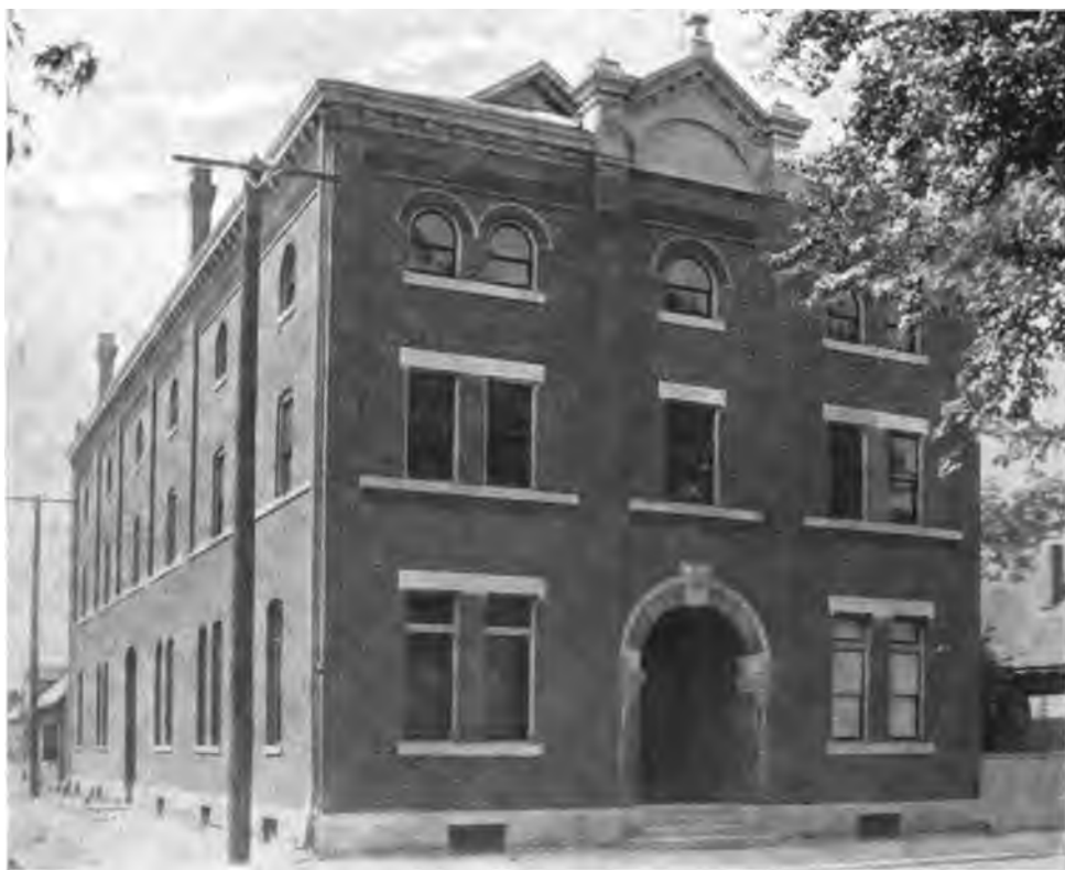
ST. JOSEPH'S HALL, INDIANAPOLIS.
